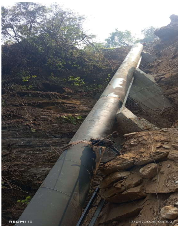
Figure 21: Installation pipe, saddle support and anchor block at vertical section.
