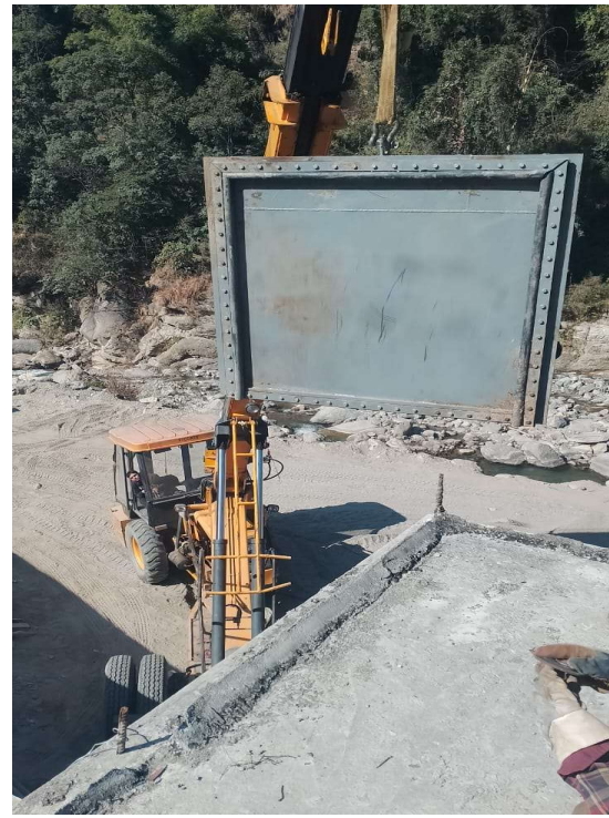
Figure 25: Gate and hoisting installation work.
