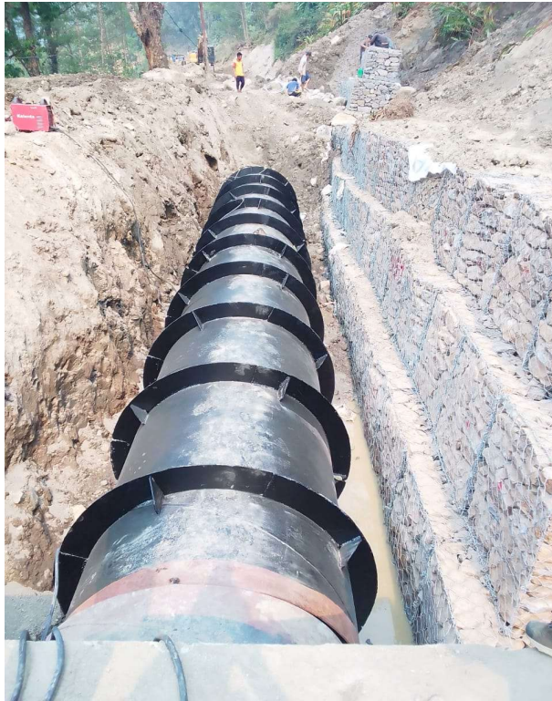
Figure 20: Pipe Installation and protection work.
